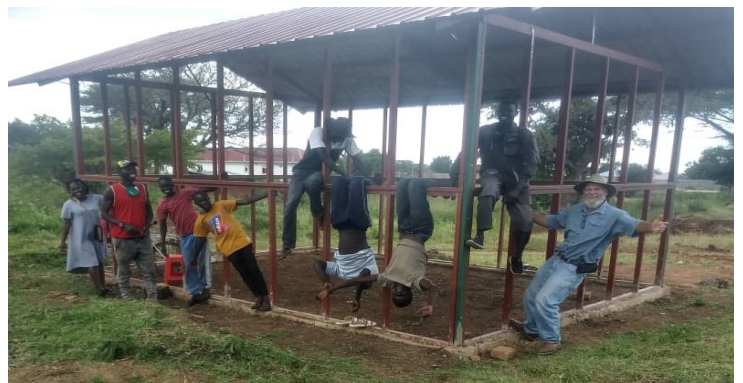
Waffle with his welding team, working on village church designs.
